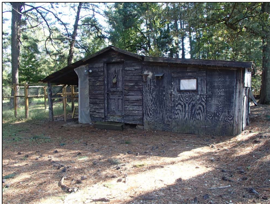
Figure 77: Bailey Tenant Farm, outbuilding
