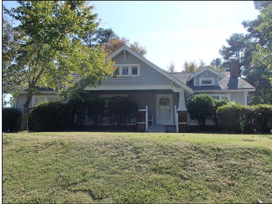
Figure 33: Sherron House, north elevation
