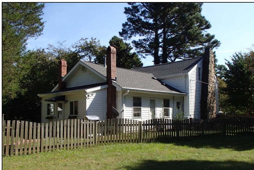
Figure 47: Sherron House, northwest corner
