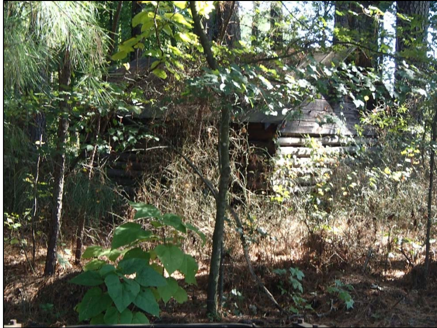
Figure 80: Bailey Tenant Farm, log crib
