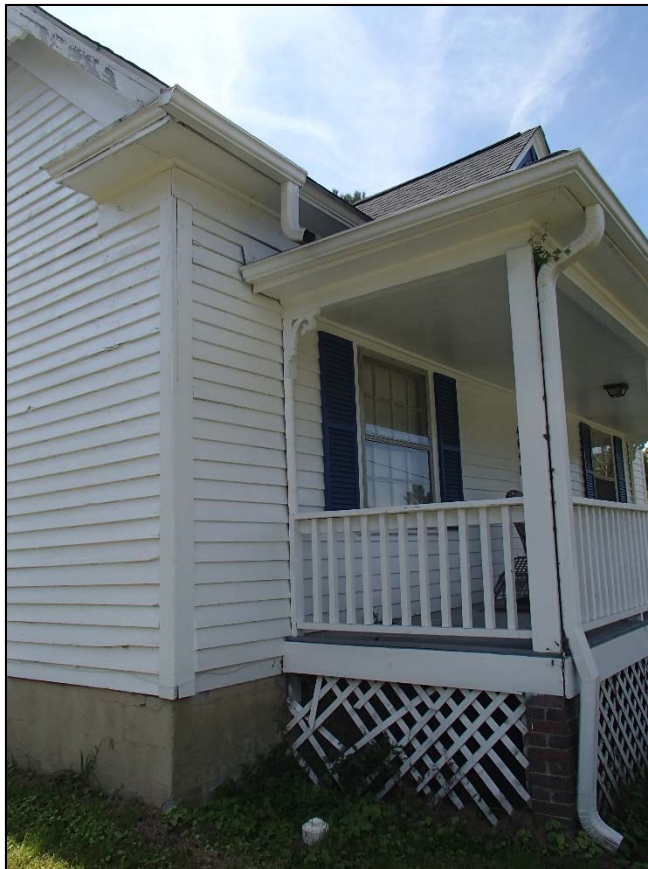
Figure 10: May House, porch detail
