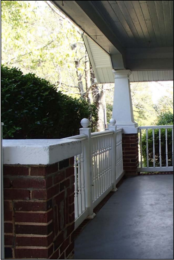
Figure 36: Sherron House, porch detail
