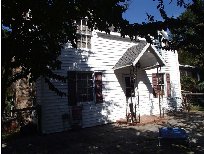
Figure 50: Sherron House, south elevation
