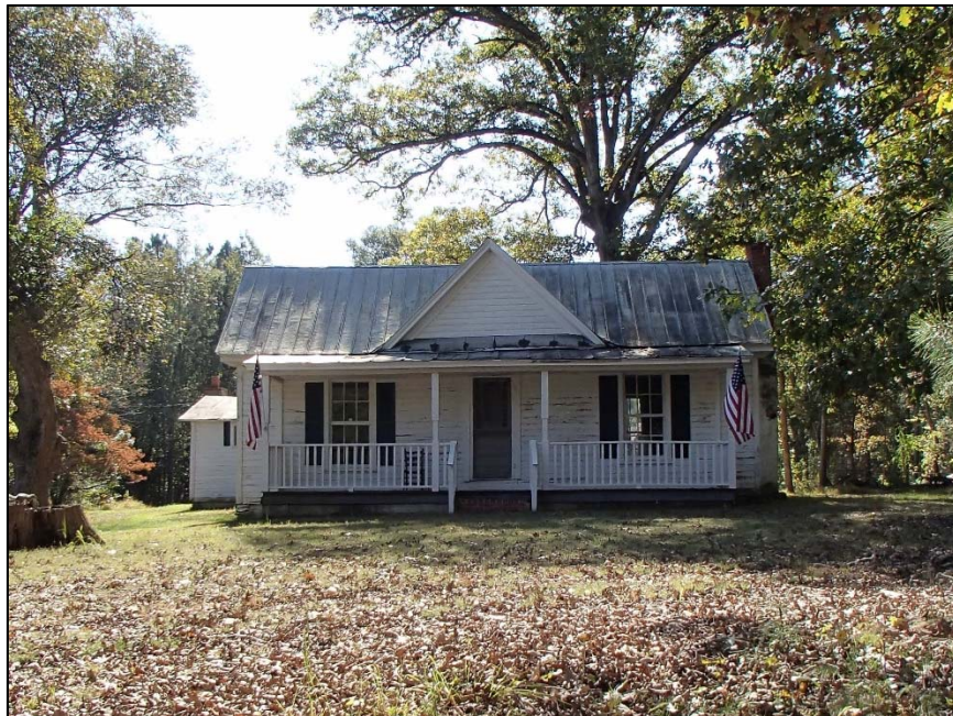
Figure 19: Poole-Terry House, DH 2521, Guess Road, with replacement porch materials
