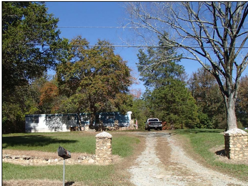
Figure 107: Wall and porch remnants at 1215 Bahama Road
