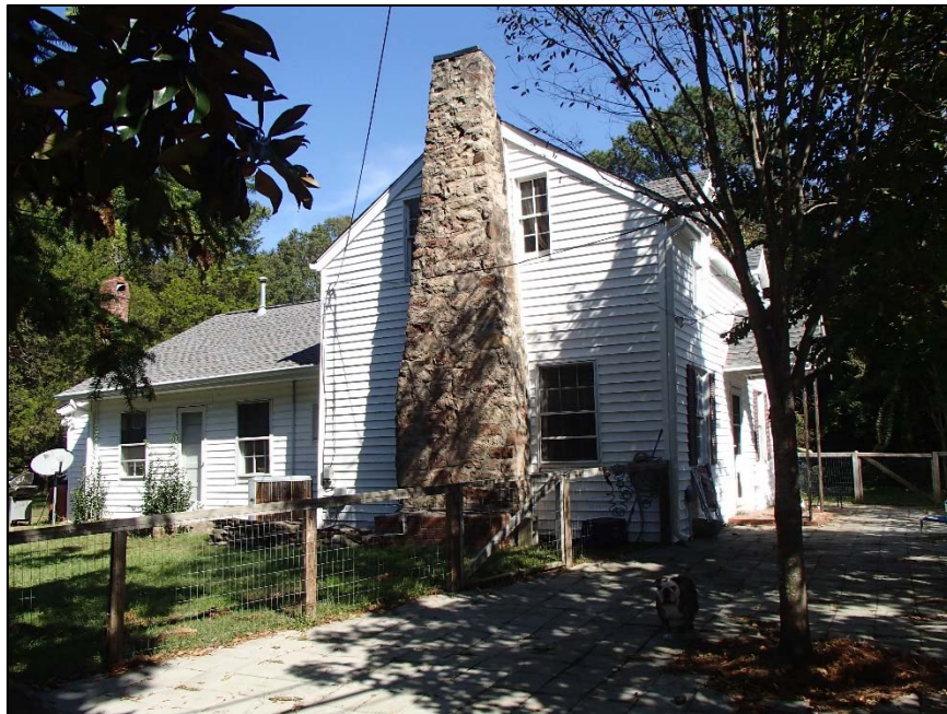
Figure 49: Sherron House, west elevation
