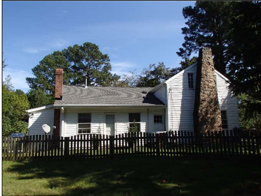
Figure 48: Sherron House, west elevation
