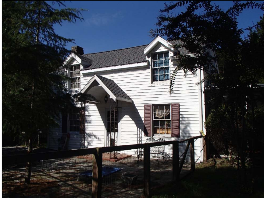
Figure 44: Sherron House, south elevation
