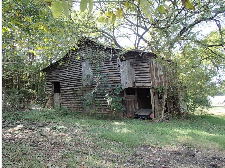
Figure 28: Beasley House, barn
