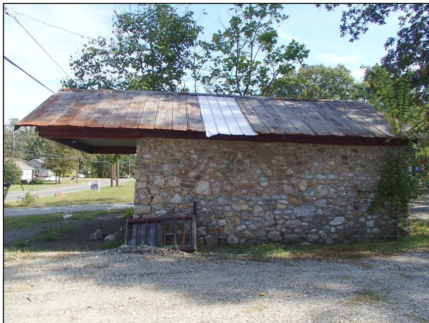
Figure 25: Beasley Store, west elevation
