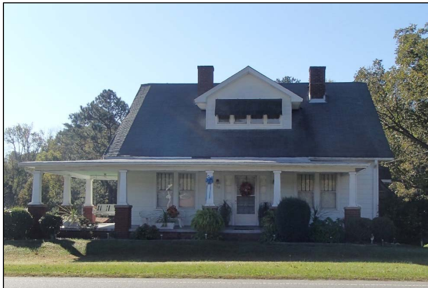
Figure 39: Bungalow at 5322 N.C. Highway 98, with vinyl siding, but retaining other original features
