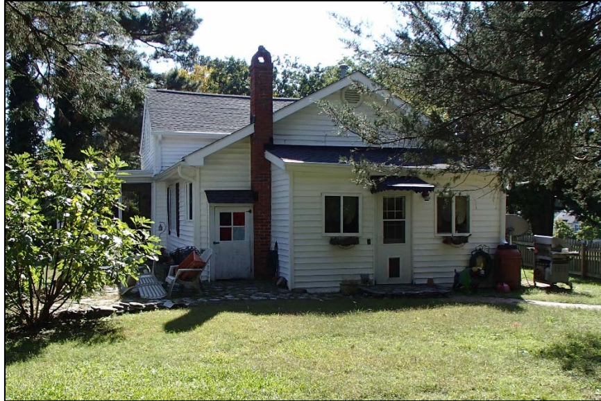
Figure 46: Sherron House, north elevation
