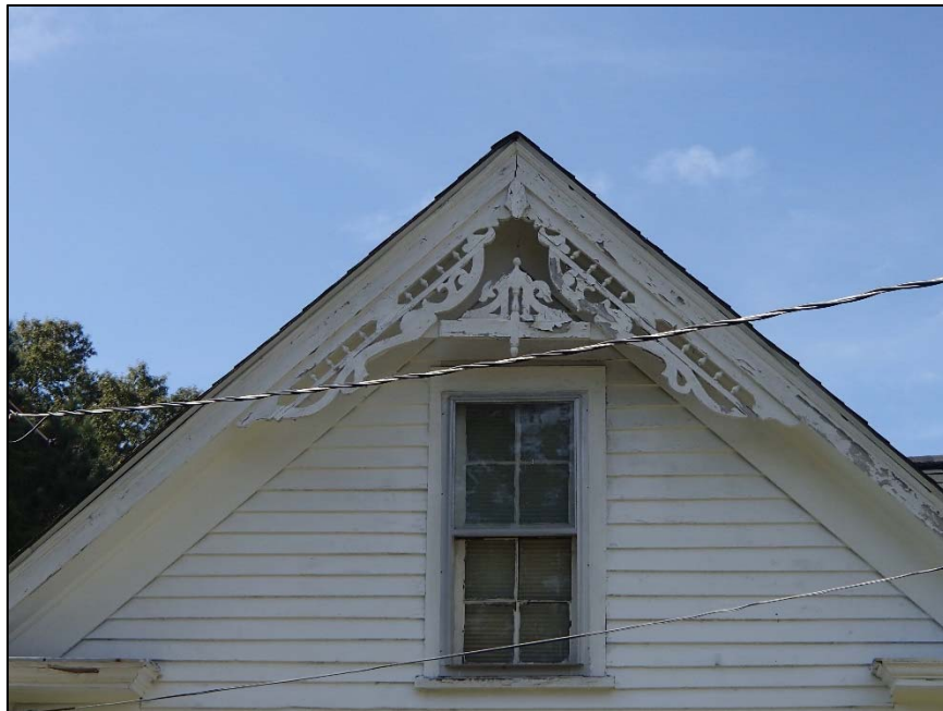
Figure 8: May House, east elevation detail
