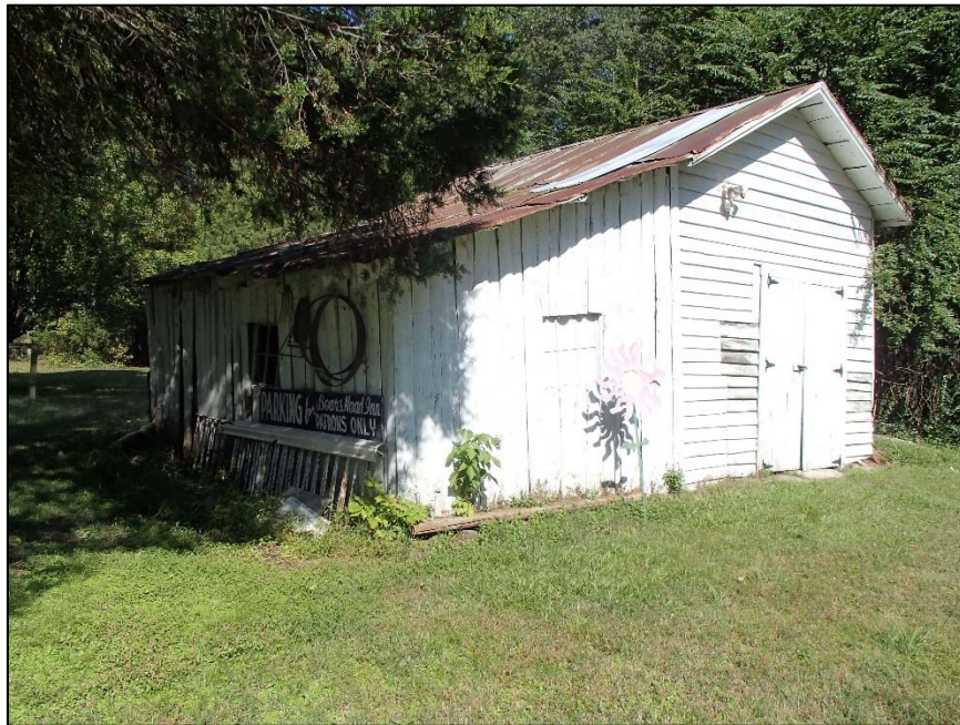
Figure 53: Sherron House, outbuilding
