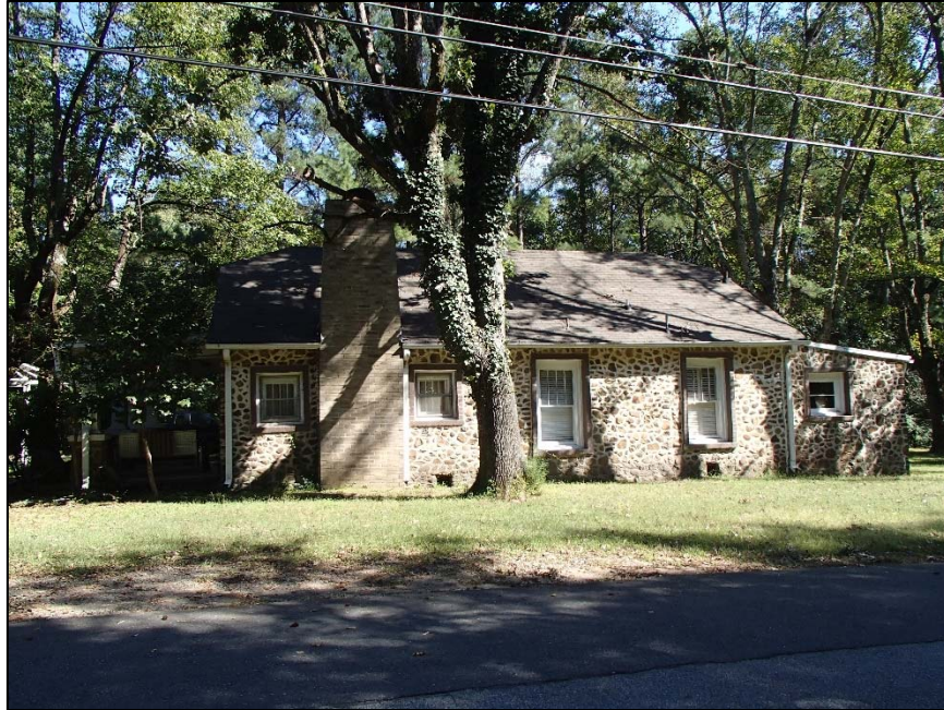
Figure 100: Choplin Place House, west elevation
