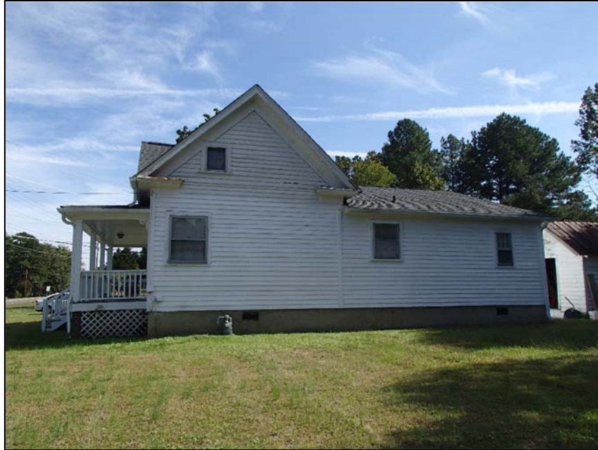
Figure 7: May House, west elevation
