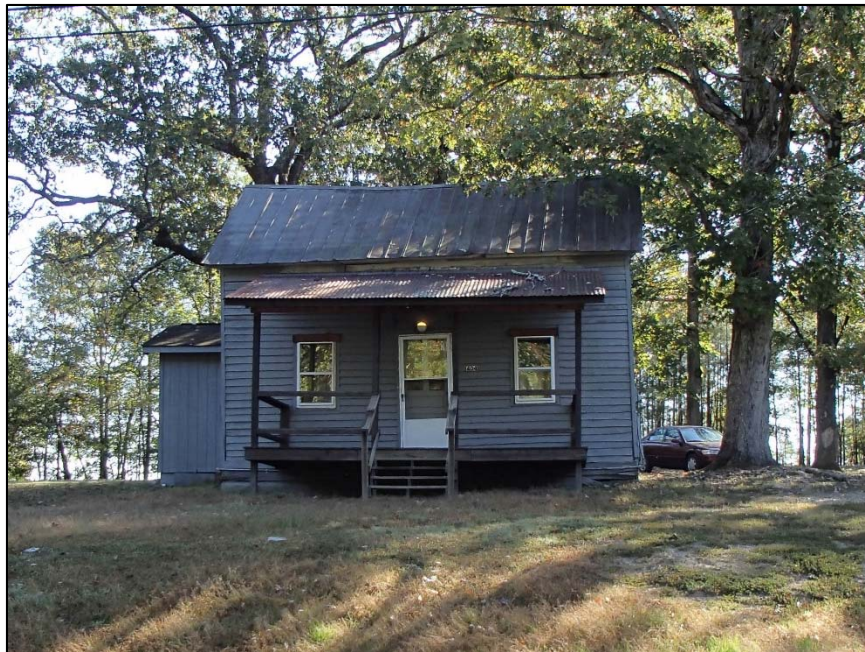
Figure 92: House at 1401 Stallings Road
