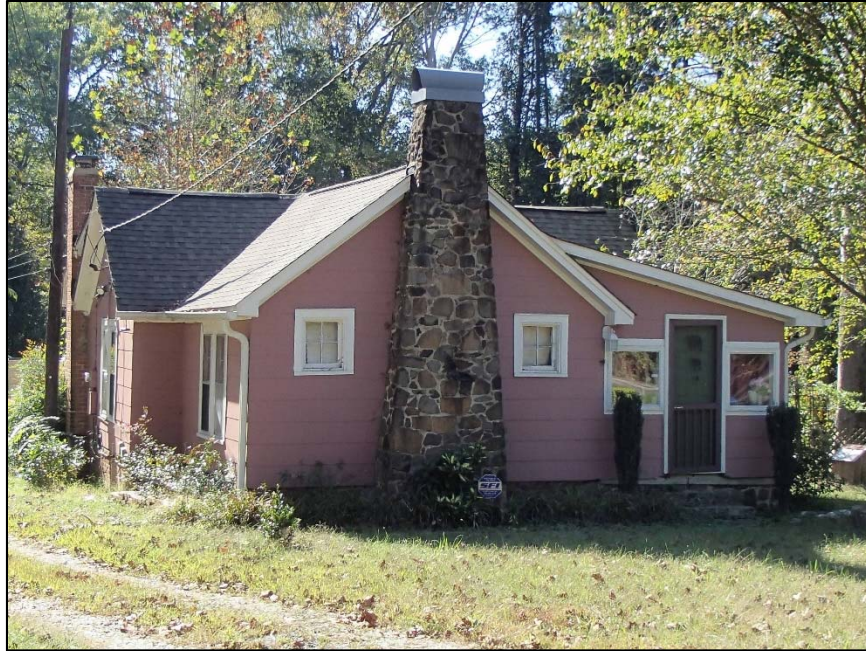
Figure 106: Chimney at 1110 Hamlin Road
