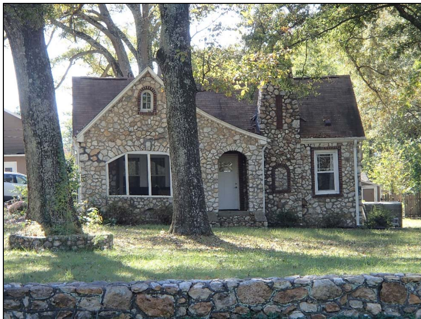
Figure 103: House at Geer Street and Watson Road
