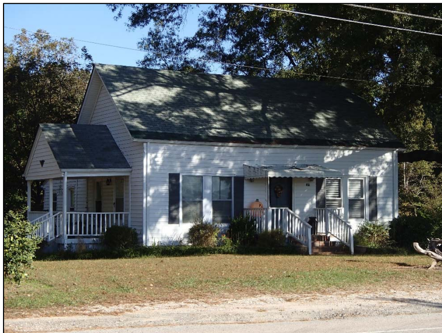
Figure 30: H. O. Carpenter House and Store, DH 2216, Baptist Road
