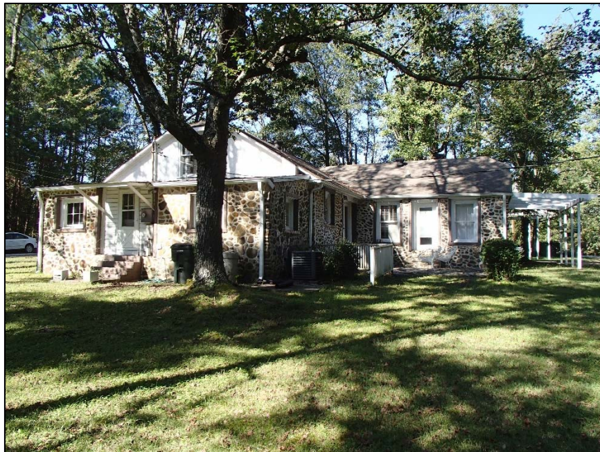
Figure 101: Choplin Place House, south elevation
