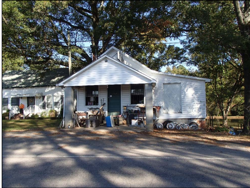
Figure 31: H. O. Carpenter House and Store, DH 2216, Baptist Road
