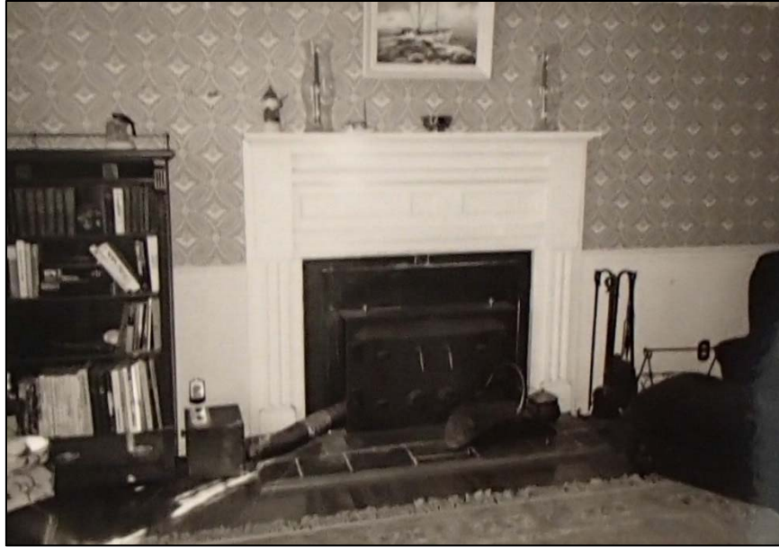
Figure 69: Coggin House, interior, 1988 survey photograph
