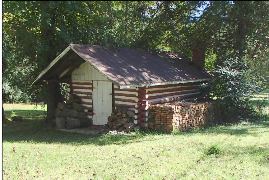
Figure 102: Choplin Place House, log outbuilding
