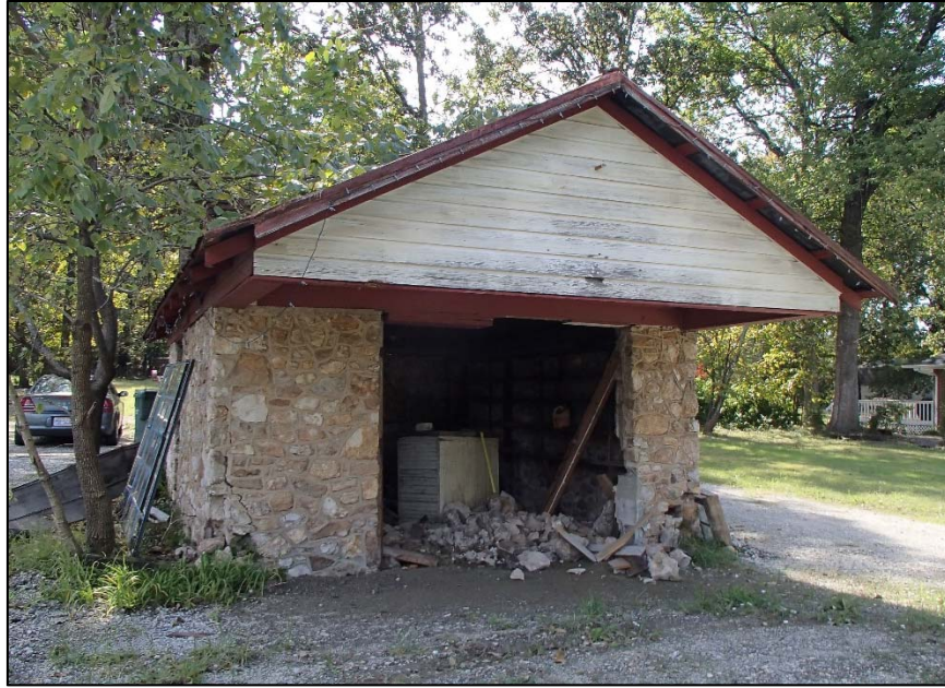
Figure 24: Beasley Store, north elevation
