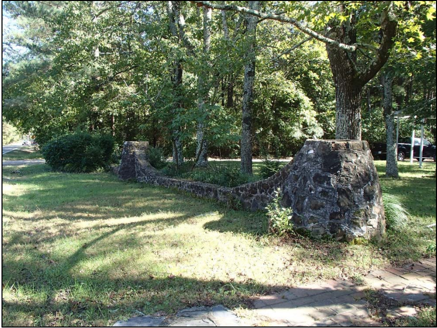
Figure 98: Choplin Place House, wall
