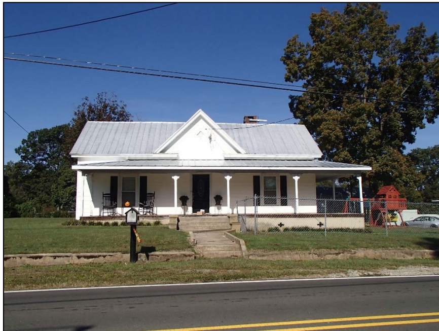
Figure 15: Copley Crabtree House, DH 2251, 1501 Bahama Road, with original porch posts, vinyl siding, and replacement windows
