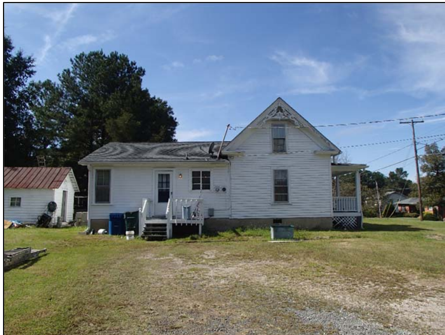
Figure 6: May House, east elevation
