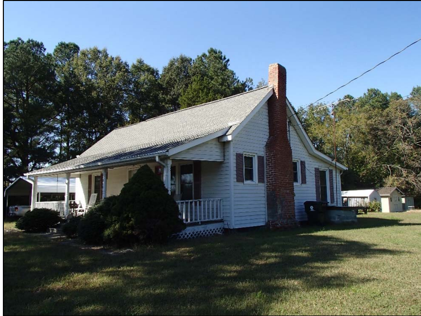
Figure 90: Rich-Yates House, southeast corner, with modern storage buildings behind
