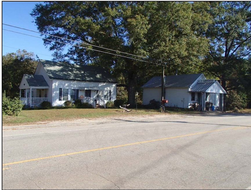
Figure 29: H. O. Carpenter House and Store, DH 2216, Baptist Road
